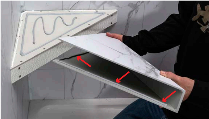
Apply adhesive just inside the edge of the bottom of the bench.
