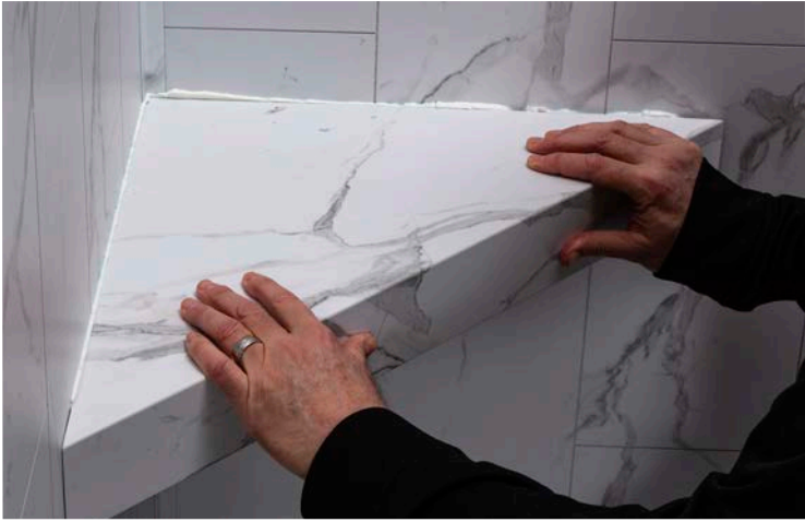
Wipe off any excess sealant that pushes out or add sealant in areas needed.
