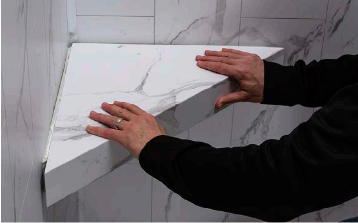
As you get closer to it being all the way in place, the sealant should start to push up to fill in between the wall and bench edge.
