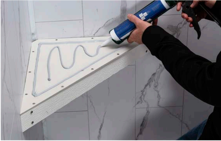
Apply adhesive to the sub-deck surface.
