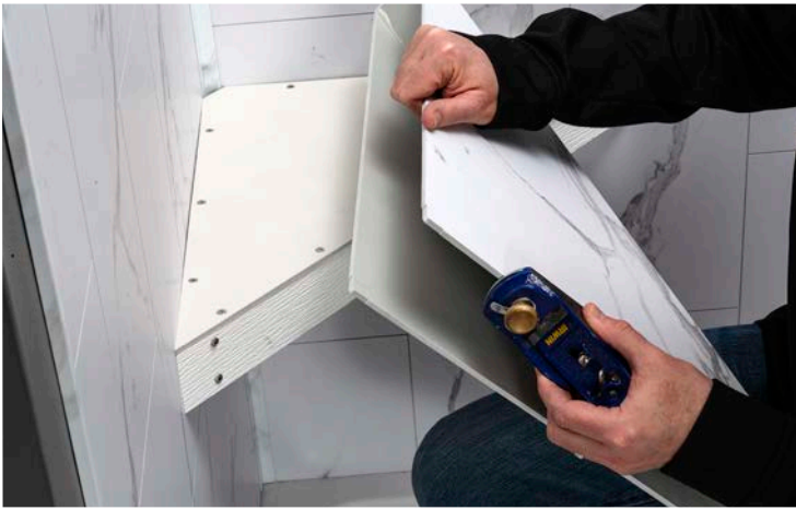
Use a plane and/or sand it to adjust the fit. Keep in mind you will need to adjust both the top and bottom of the bench.
