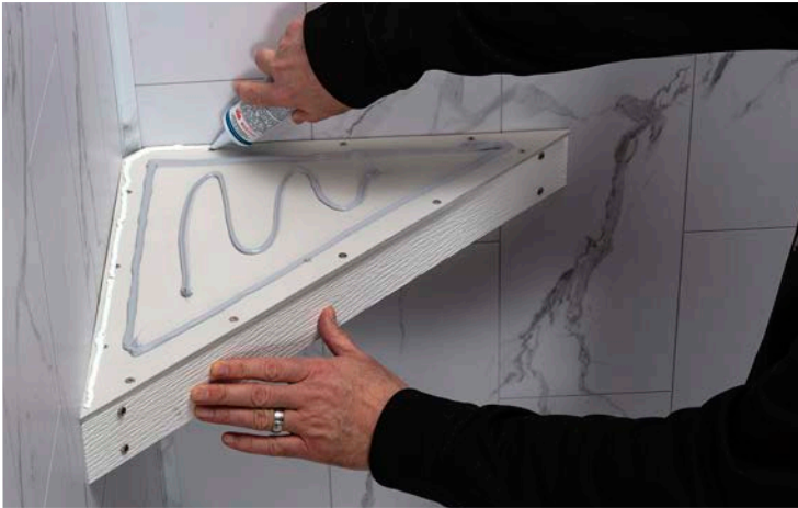
Apply a bead of sealant where the wall and sub-deck meet.
