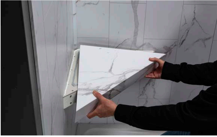
Carefully slide the bench into place.
