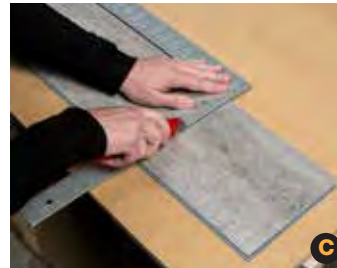
Cut Palisade planks by scoring and snapping with a utility knife. (image C, D). This method may require sanding the snapped edges.
