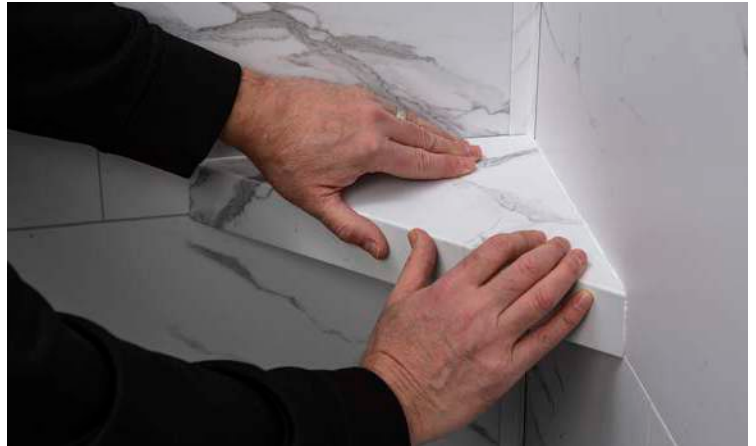
Wipe off any excess sealant that pushes out or add sealant in areas needed.
