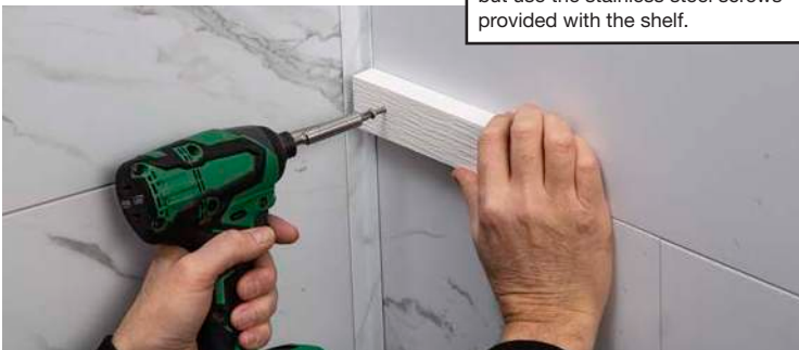
Install the first screw closest to the corner of the shower.
