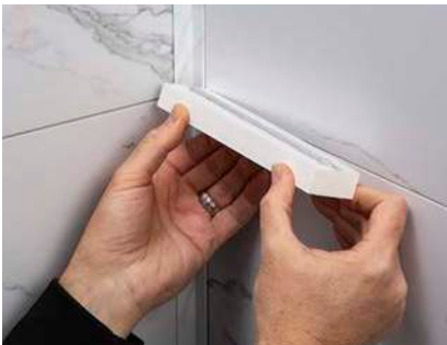
After locating where you want to place the shelf, put adhesive onto bracket.
