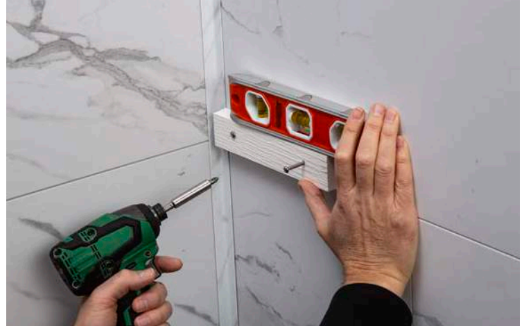
Before installing the second screw, be sure to level the bracket.
