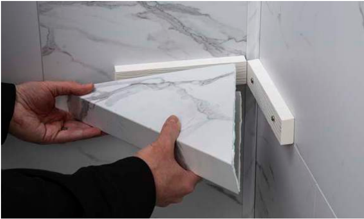
Carefully slide the shelf onto the brackets.
