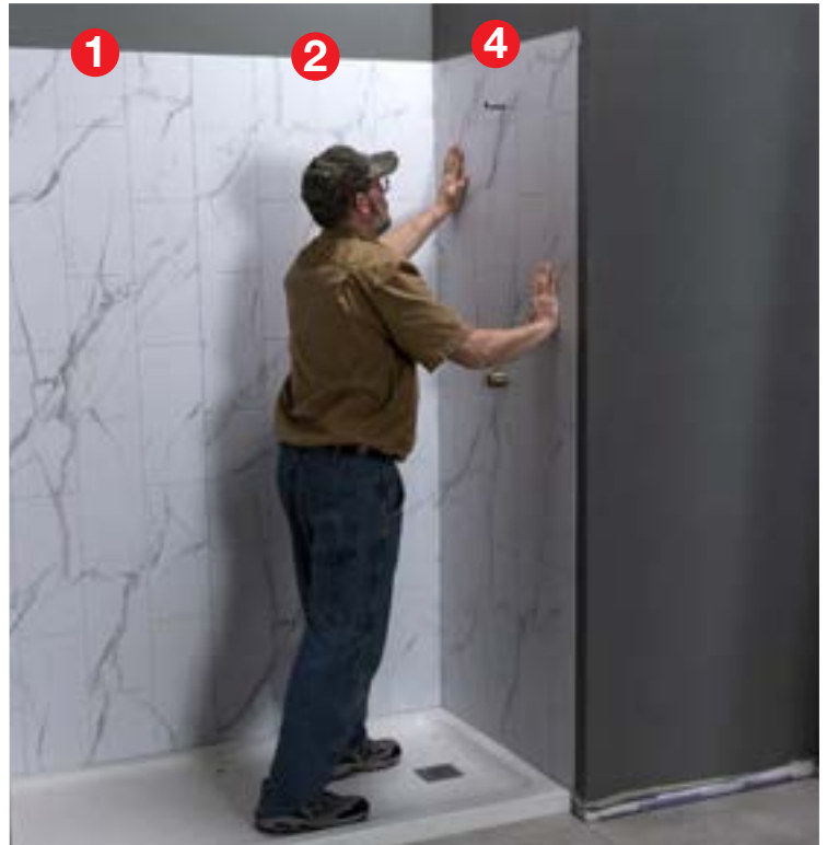
Also make sure it is fitting nicely to the plumbing.
