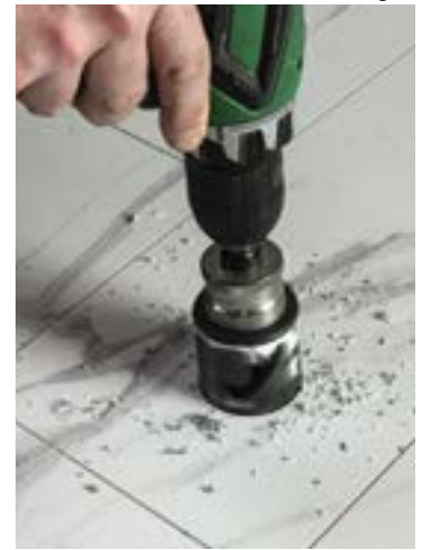
Cut panels to accommodate shower components. Measure and mark the locations and use one of these types of drills or hole saws.
