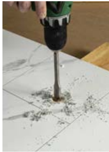
Cut panels to accommodate shower components. Measure and mark the locations and use one of these types of drills or hole saws.
