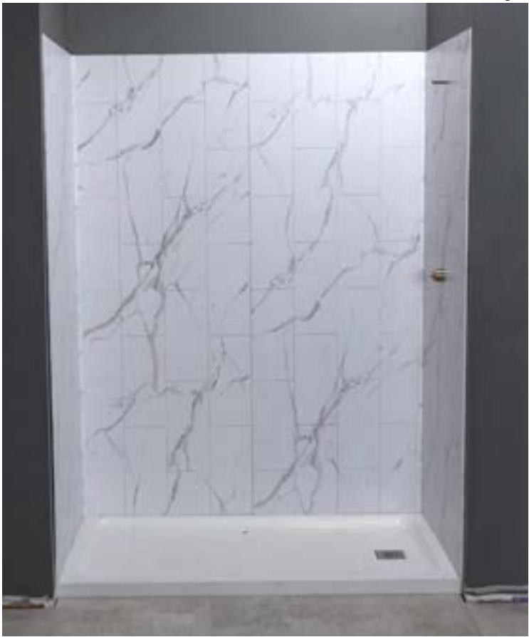
Completed shower wall system install.
