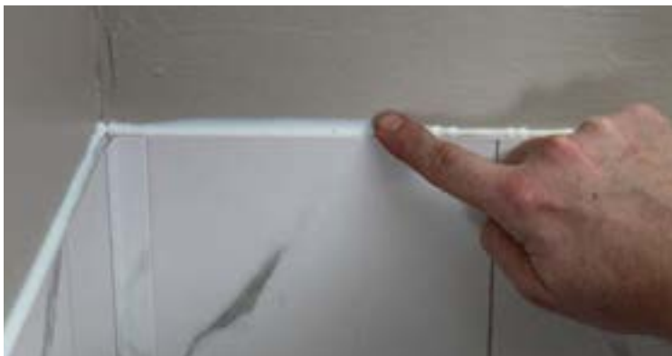
Smooth the sealant across the panels for adequate coverage.
