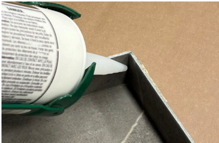
Apply 100% silicone along the vertical seams in each inside corner. See detail below.
