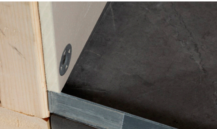
Waterproof wallboard installed prior to curb installation.
