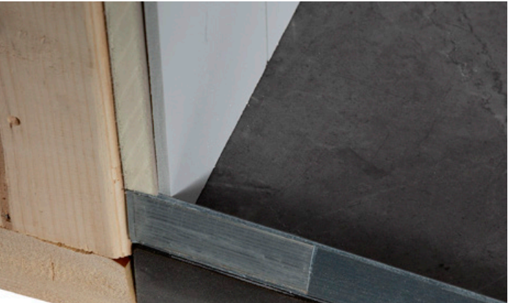
Waterproof wallboard and PVC shower wall panels installed prior to curb installation.
